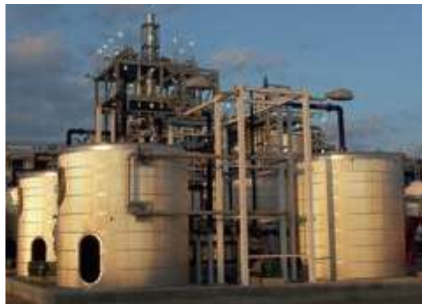
A simulated moving bed chromatography system for manufacture of an organic acid (with permission from Escon GmbH)
